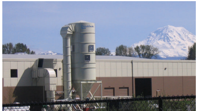
528LP12 at Cabinet Factory 70,000 cfm (118,906 m 3 /h)
